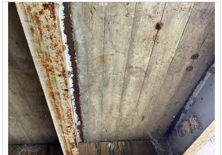
Bay 5 in between girders 4 and 5 has minor cracking with efflorescence.
