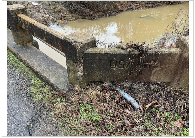
Spalling in bridge railing left and right sides.
