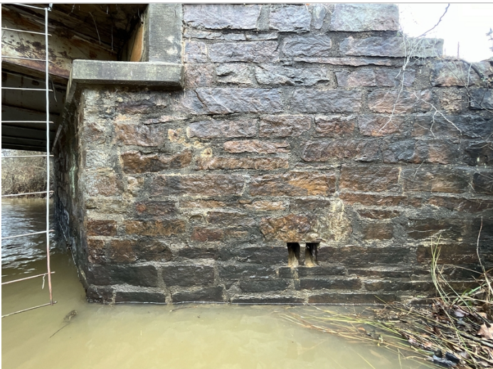
Minor cracking with efflorescence in the wing wall.
