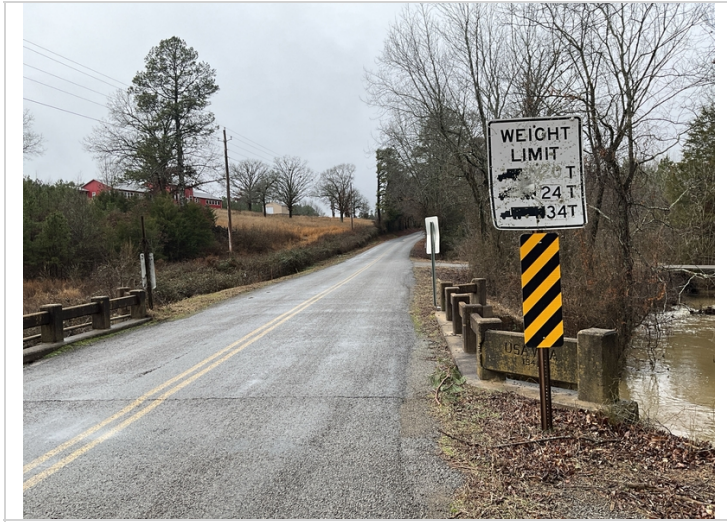
Load posting sign is damaged
