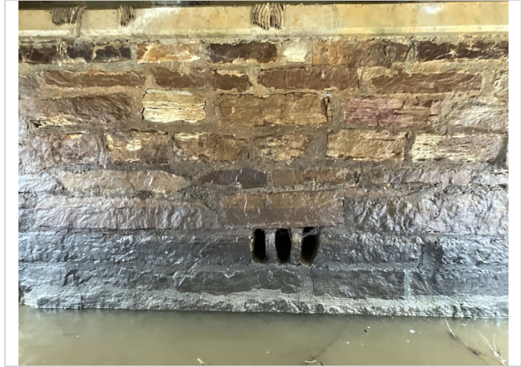
Cracking and mortar break down in abutment 2.
