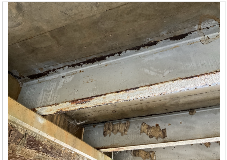
Minor rust on beam ends.
